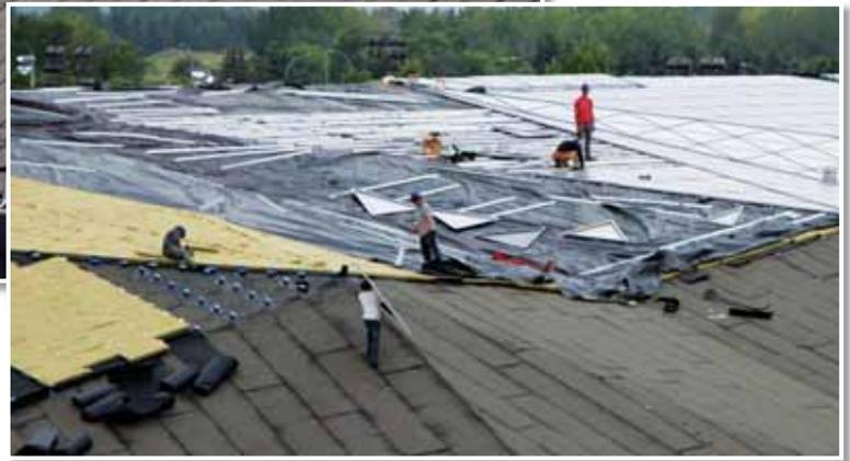
By completion of the project, Skyline Roofing will have removed and refurbished 12,000 triangular panels and re-installed them in their original location.
